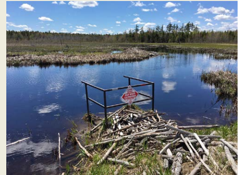
Above: Aged DUC water control structures in need of replacement at (top to bottom) Jack Pine Meadow and Shirley's Meadow.
